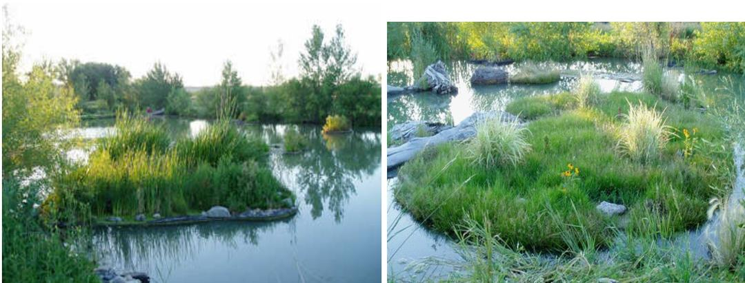
Figure 3 Example of constructed floating islands deployed in small ponds for habitat and treatment benefits.
